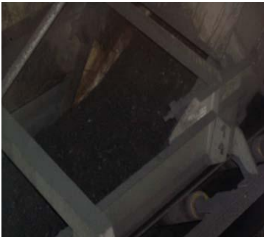
Figure 4: Guides at the edges of Conveyor Belt to avoid Spillage
