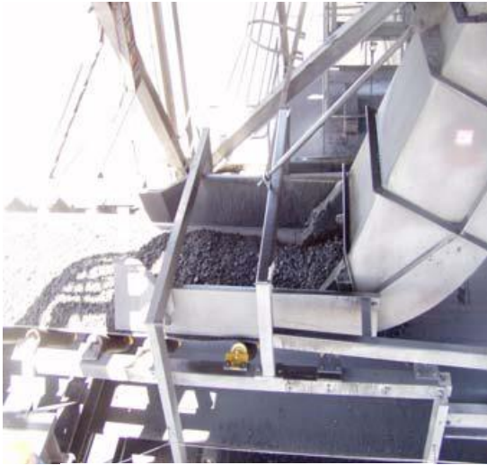
Figure 3: Covering inclined section of Conveyor
